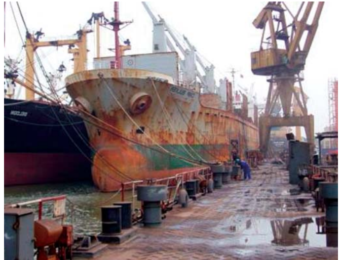
Ship under repair at Wenchong Shipyard
