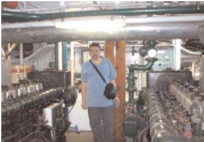
David at work in the engine room on Bounty
