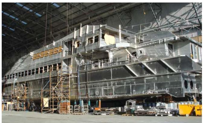
Vessel under construction in shed
