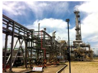
Part view of the chemical processing plant
