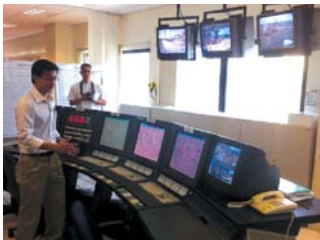
Control room of the training centre
